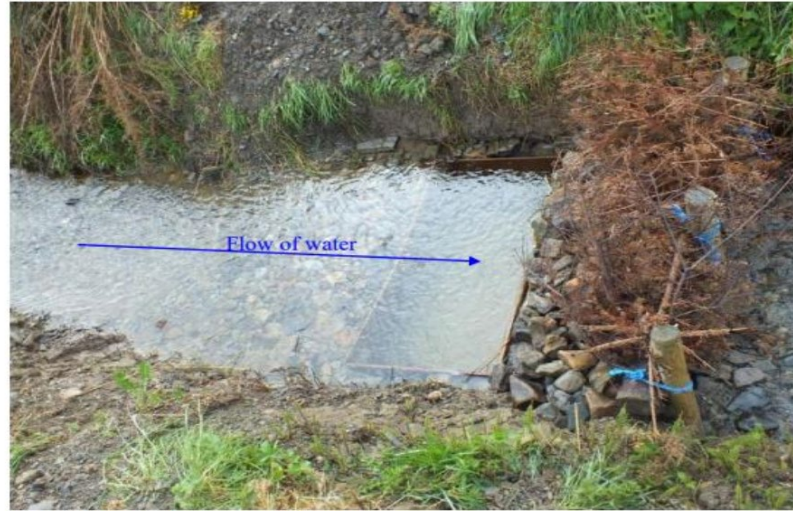
Figure 7 Silt trap installed in stream at Kilberriert
